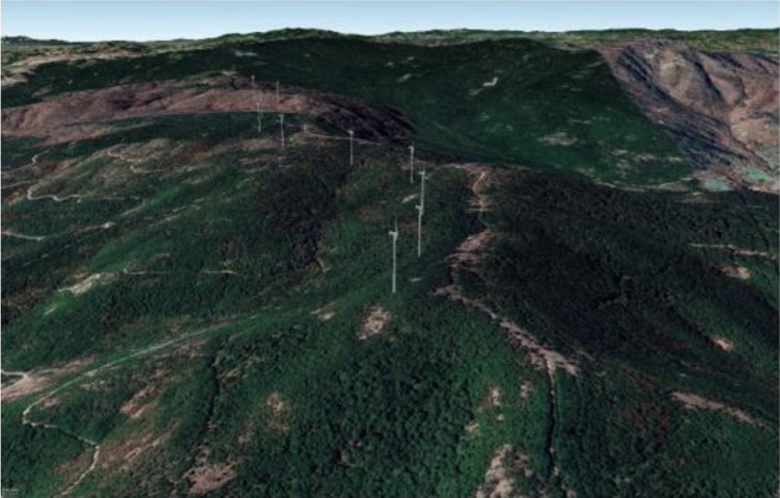
Picture 19: Panoramic view of the WPP with shooting direction west
